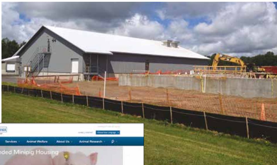
Construction of our new minipig barrier is underway.
