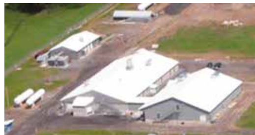
Barrier Breeding Facility Today with New Addition
